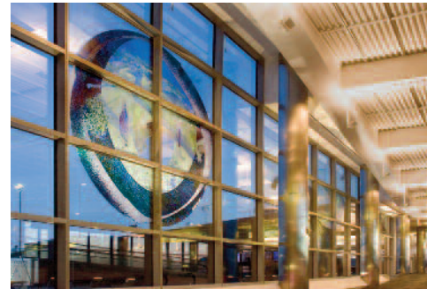
BWI/Thurgood Marshall Airport
